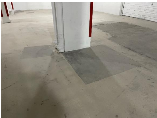
Photo 5: Concrete repairs at underground parking garage.
