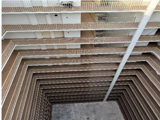
Photo 7: Inside, exterior walkways at North side.
