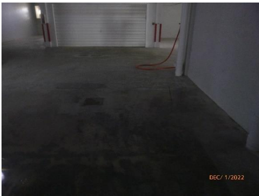
Photo 3: Concrete repairs at underground parking garage.
