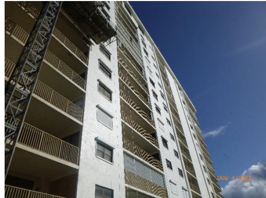
Photo 2: South side of the building.
