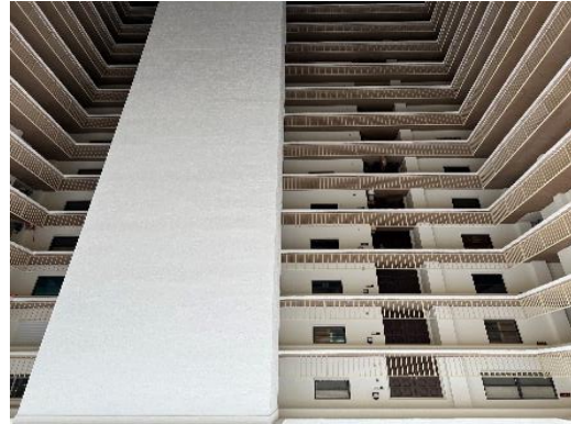
Photo 8: Inside, exterior walkways at East side.
