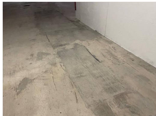
Photo 6: Concrete repairs at underground parking garage.
