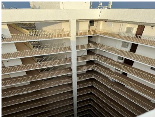
Photo 9: Inside, exterior walkways at South side.
