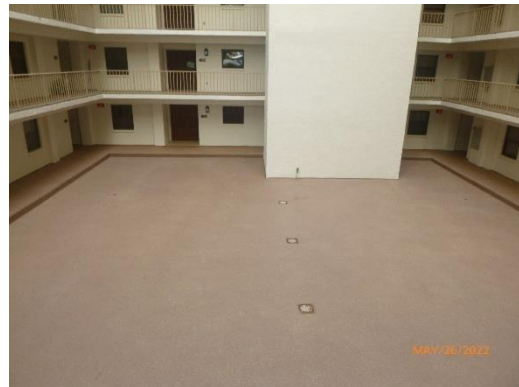
Photo 12: Deck coating installed at atrium.
