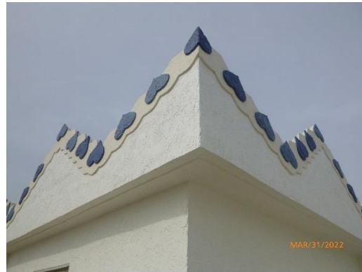
Photo 14: Painted roof structure.
