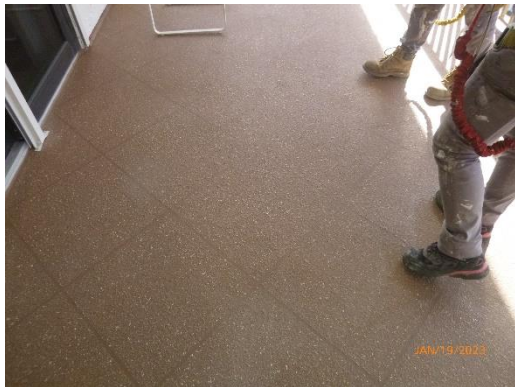
Photo 11: Balcony with replaced deck coating.
