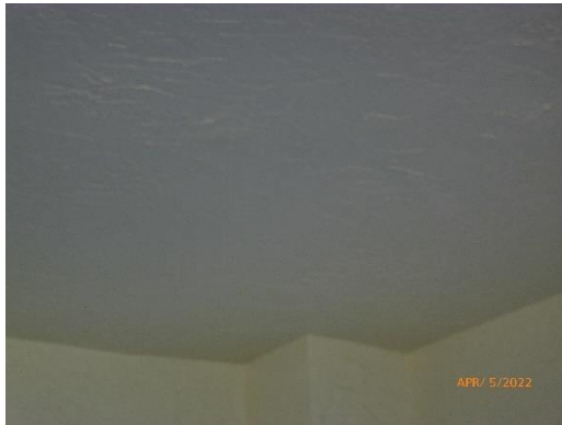
Photo 13: Painted ceiling at balcony.
