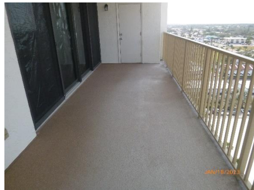
Photo 10: Balcony with replaced deck coating.
