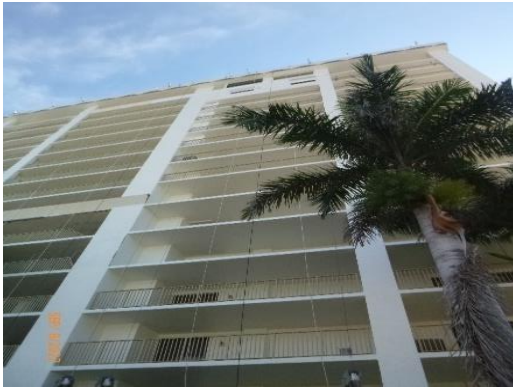
Photo 1: West side and front of the building.
