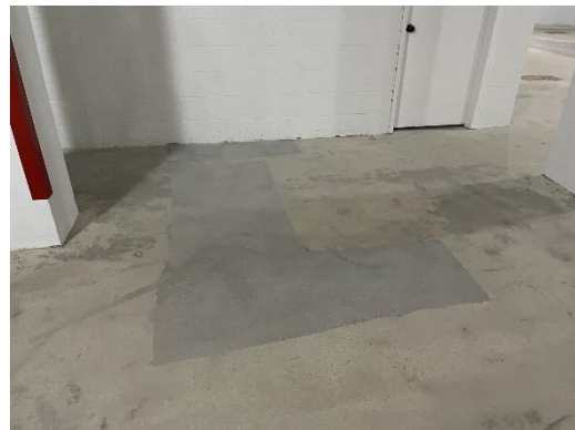
Photo 4: Concrete repairs at underground parking garage.
